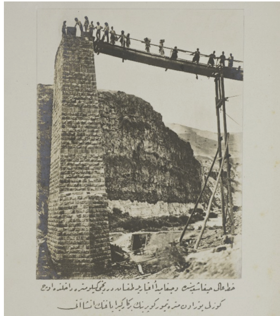
Figure 2. "The Haifa branch of the Exalted Line and construction of the stone column at the beginning of the three arched 110-meter-long railway bridge at the 94th kilometer of the Haifa branch" ( hat-ı ali Hayfa şubesinde ve Hayfa mebde itibarıyla doksan dördüncü kilometre dahilinde üç gözlü yüz on metre demir köprüünün bir kargir ayağının inşası ) shows workers on top of the temporary wooden bridge connecting the two main stone pillars of the bridge over the river in the Haifa branch of the Hijaz Railway. Source: Ömer M. Koç Collection.
